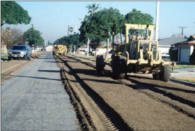
Figure 3.3 Grading and shaping.
