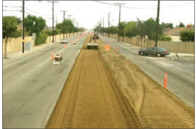
Figure 3.10 Traffic control in an urban area.
