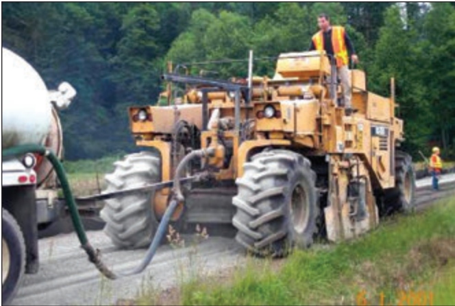
Figure 3.7 Water being injected during mixing operation.
