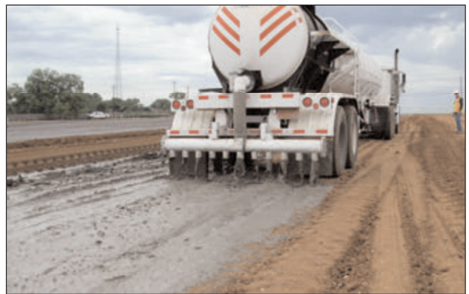
Figure 3.5 Placing cement in slurry form.
