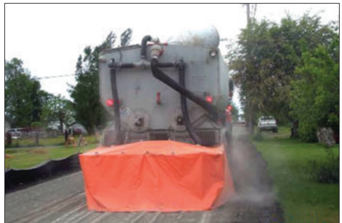
Figure 3.6 Enclosure for dry cement application.
