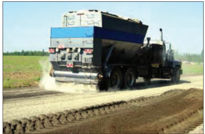
Figure 3.4 Placing cement dry.
