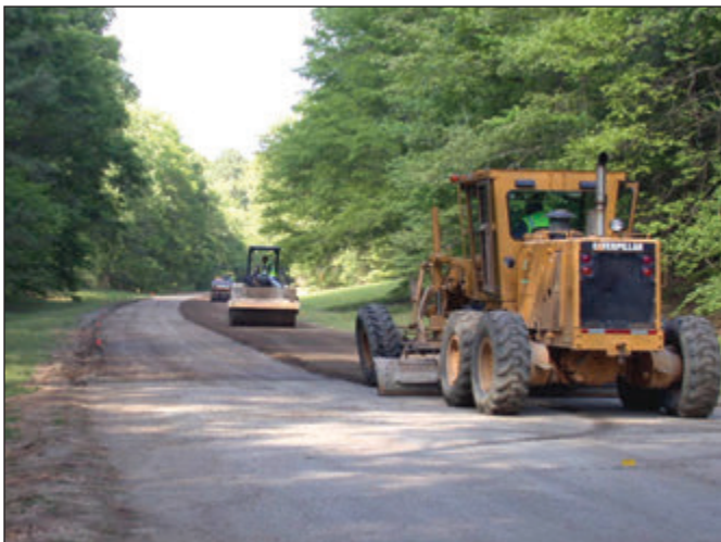
Figure 3.8 Compaction and final grading.
