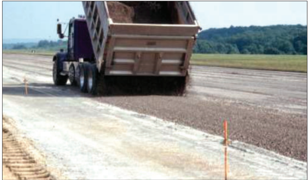
Figure 2.2 Placing additional aggregate for inclusion in the FDR process.
